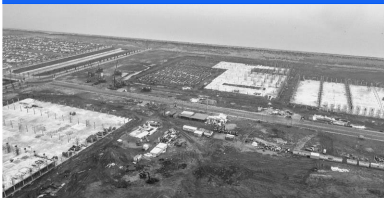
2017 – Company Founding and Facility Construction
